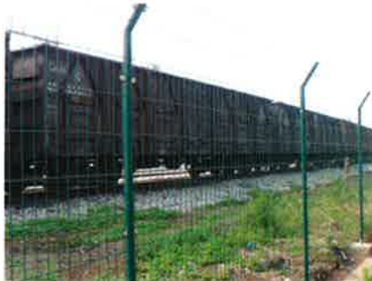
Rail Security Fence
